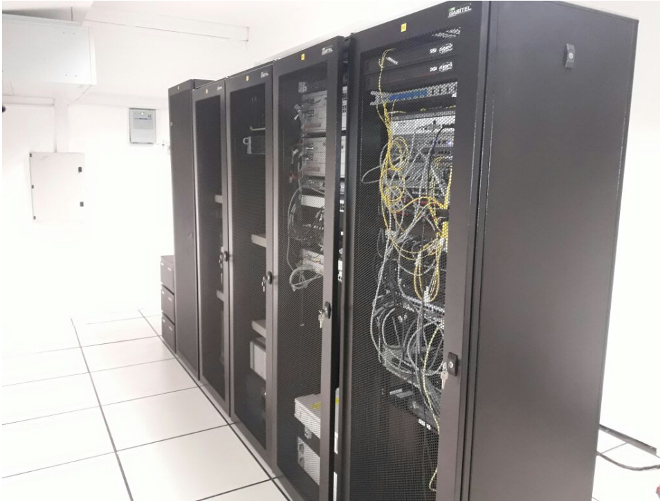
Figure 21 -Existing Data Center Equipment (Cabinets)
