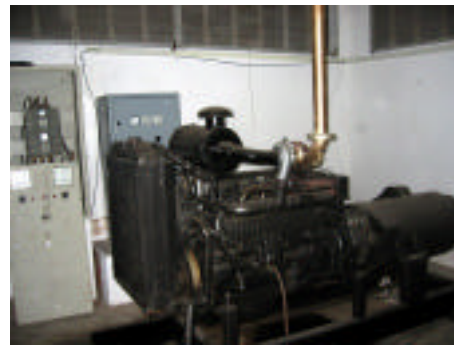
Backup generator for data center and Telemar-operated NOC
